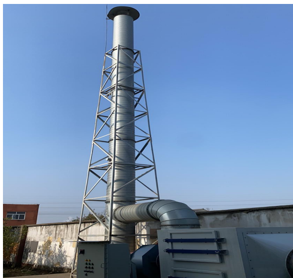
涂料生产废气 15m 排气筒
